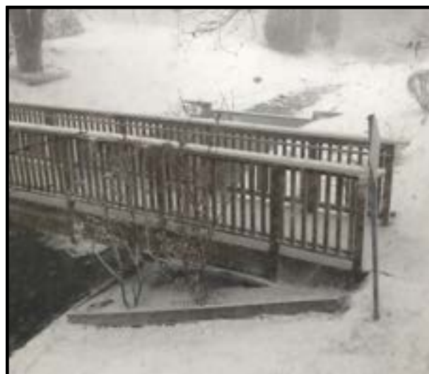
Sikwan: Looks like winter still – but under the bridge the ice has melted.
